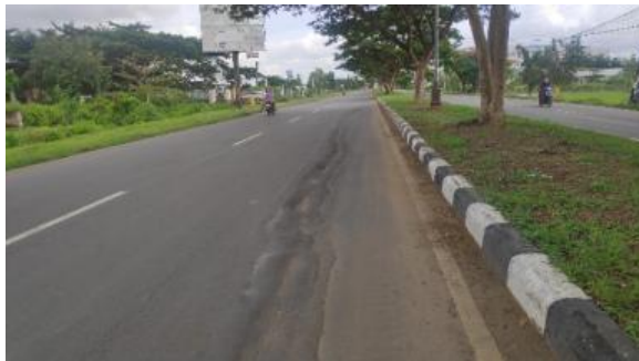
Figure 14. Lightly damaged road (Unsatisfactory)
